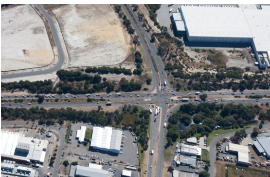
Before: Tonkin Highway/Horrie Miller Drive/Kewdale Road
