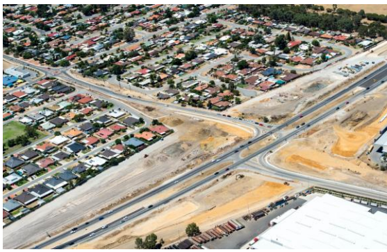
Early construction: Roe Highway/Berkshire Road
