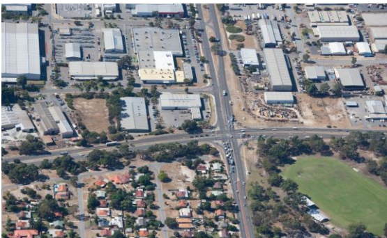
Before: Leach Highway/Abernethy Road
