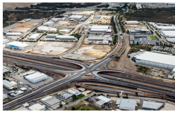
Completed: Tonkin Highway/Horrie Miller Drive/Kewdale Road
