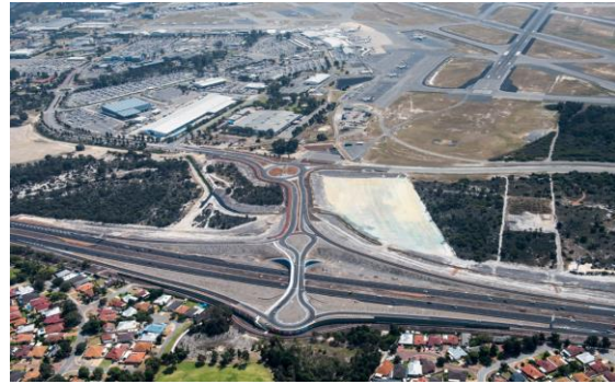
Completed: Tonkin Highway/Dunreath Drive
