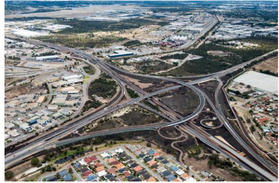
Completed: Tonkin Highway/Roe Highway
