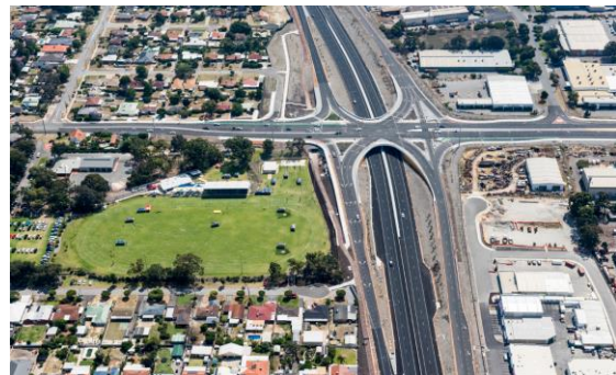
Completed: Leach Highway/Abernethy Road
