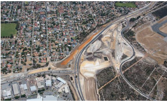
Early construction: Tonkin Highway/Leach Highway
