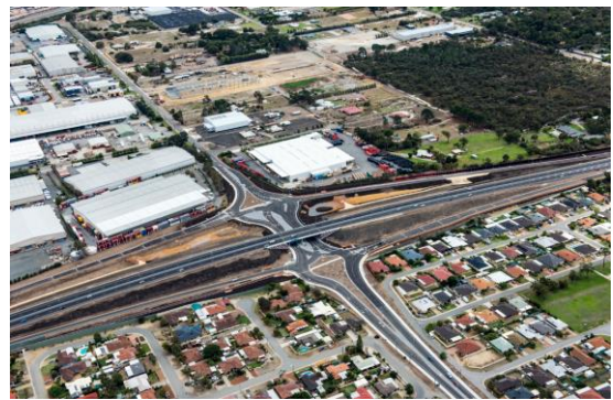
Completed: Roe Highway/Berkshire Road
