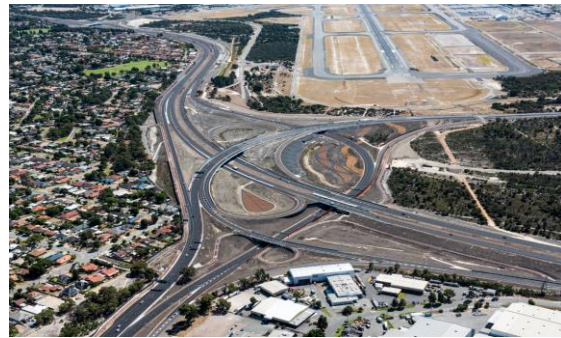
Completed: Tonkin Highway/Leach Highway
