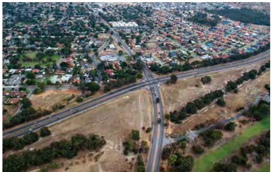
Noise / amenity walls will be constructed along the western side of Roe Highway
