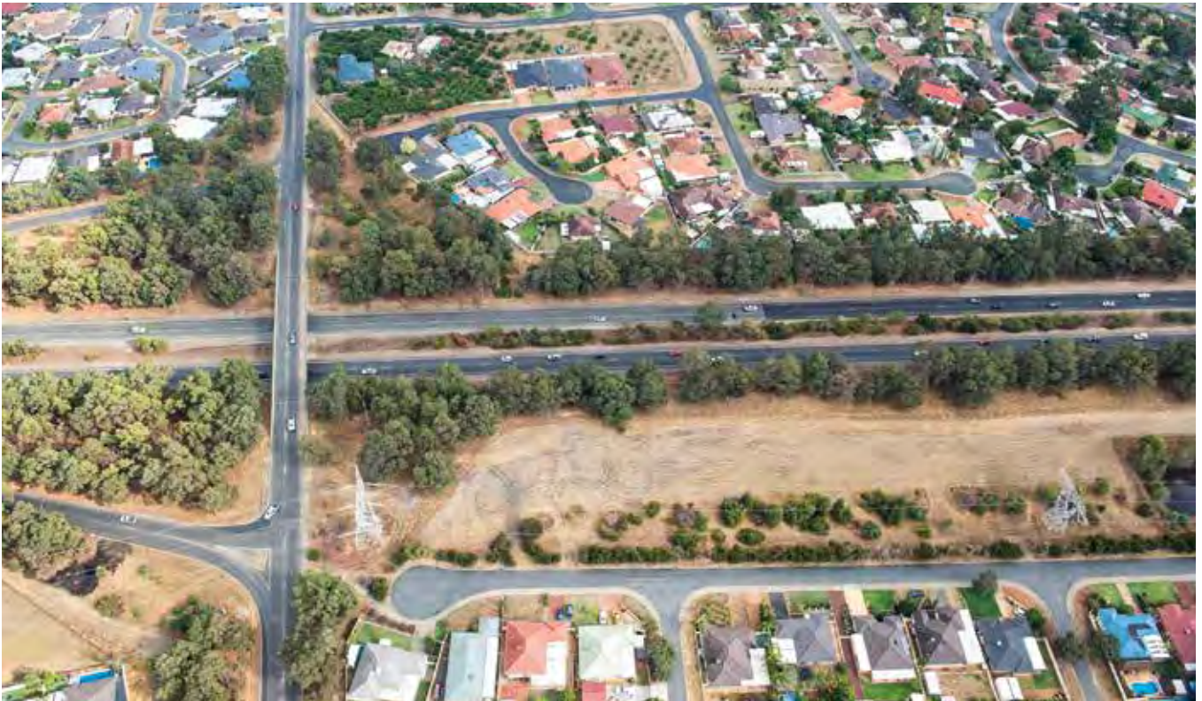
The noise / amenity walls will mitigate traffic noise and provide privacy screening for local residents
