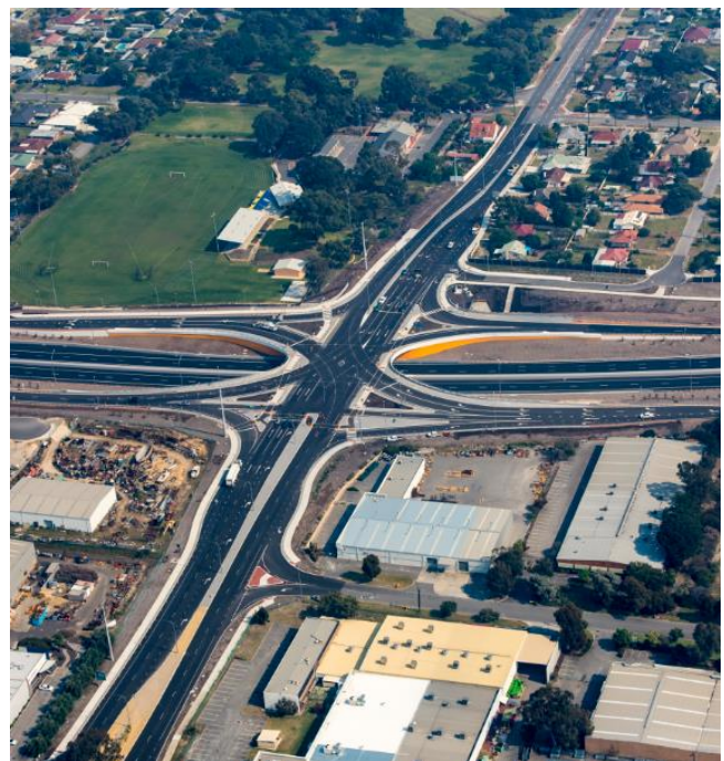
Above: An aerial photograph of the Leach Highway / Abernethy Road interchange, looking north, taken in September 2015.
